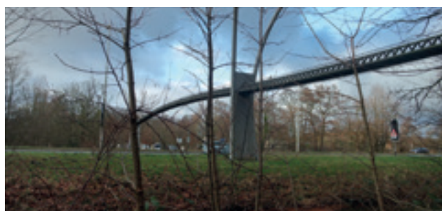
‘Eek-o-duct’ over de N44
